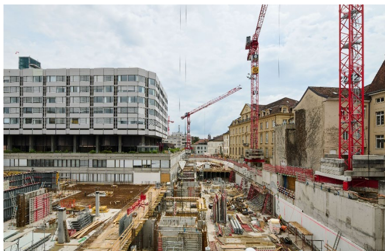
New building Clinic 2, Universitätsspital Basel (Foto: Studio-Willen)
